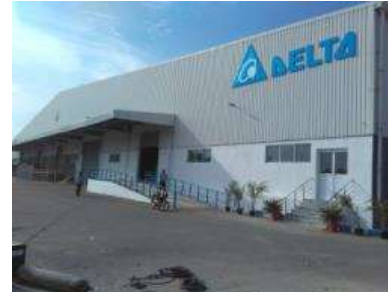
Site Front View
